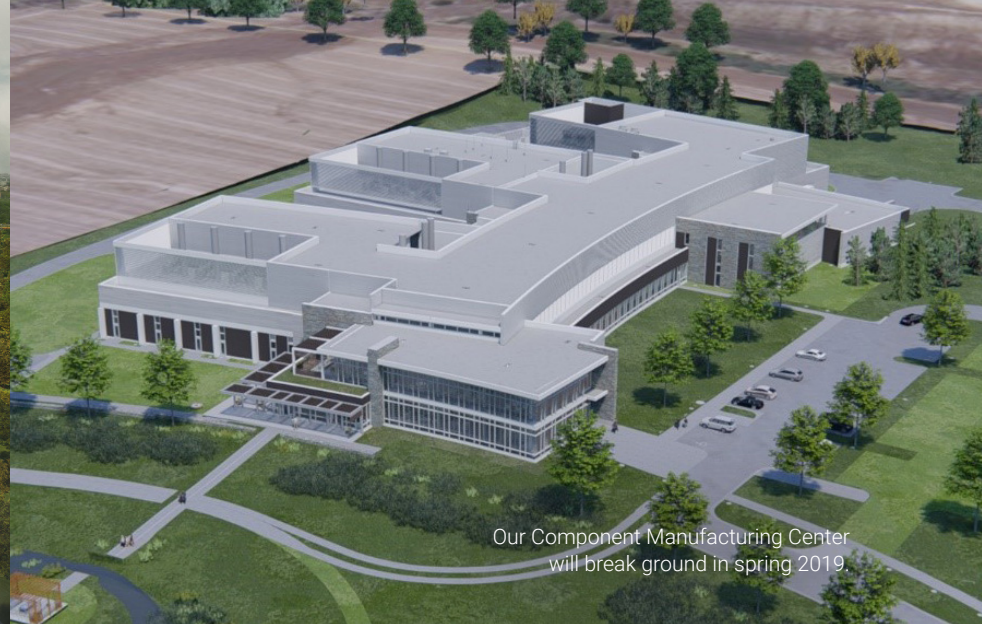
A rendering of the new Research and Development Facility being constructed in Madison, Wisconsin.
